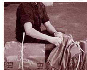
Tie straps around polyethylene encasement
