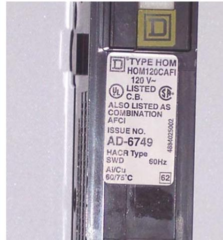
**Figures 2 & 3 – Labels Indicating Branch/Feeder and Combination Type AFCIs**
