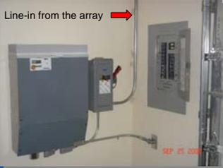
In this system the utility grid provides the back-up power and eliminates the need for batteries in the system
