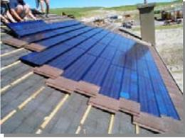
Some manufacturers of PV roofing tiles have tested their products and meet the standard for Class A roofing
