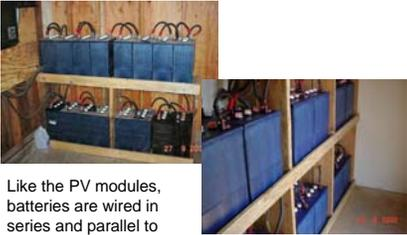
Like the PV modules, batteries are wired in series and parallel to provide the voltage and amperage necessary for the operation of the electrical system
