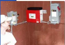
In this system the inverter is flanked by two disconnects the right disconnects the array and the left disconnects the inverter from the main electrical panel
