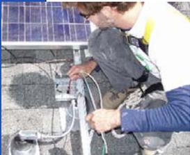
National Electric Code specifies that conductors of different output systems will be contained in separate raceways, cable trays, cable, outlet box, junction box, or similar fittings
