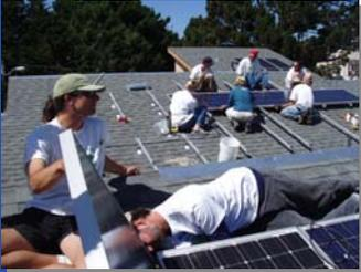
PV modules can be mounted directly on the roof, in many cases specialized roof racks lift the array from the roof deck allowing air to circulate under the modules.
