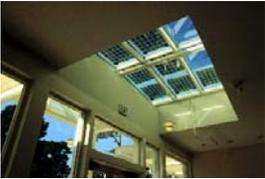
A skylight with integrated photovoltaic will have a distinctive amorphous rectangular pattern in the glass
