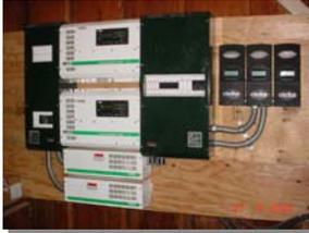
Battery charge controllers are found in off-grid systems and grid-tied systems that have a battery back-up.
