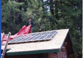
Foam will not block out all the sunlight and will slide off the array
