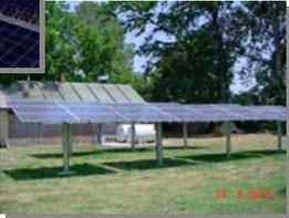
PV systems can also be mounted on the ground using customized racks, or they can be mounted on poles.
