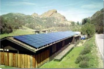
Pinnacles National Monument in California installed a 9.6-kilowatt photovoltaic system. It eliminates the fuel bill for a diesel generator that produced 143 tons of carbon.
