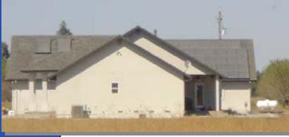
Two solar hot water panels are on the left of this roof and 44 modules of this 7 kw PV array on the right of this 3,000 sq. ft. home. The system is backed-up with a generator.
