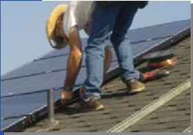
Exposed non-current-carrying metal parts of module frames, equipment, and conductor enclosures shall be grounded regardless of voltage
