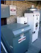
You may not be able to see a PV system on a flat roofed building from street level. The large inverters at the USPS processing and distribution center in Marina Del Rey, would be your first clue of the existence of a 127 kw monocrystalline PV system on the roof.
