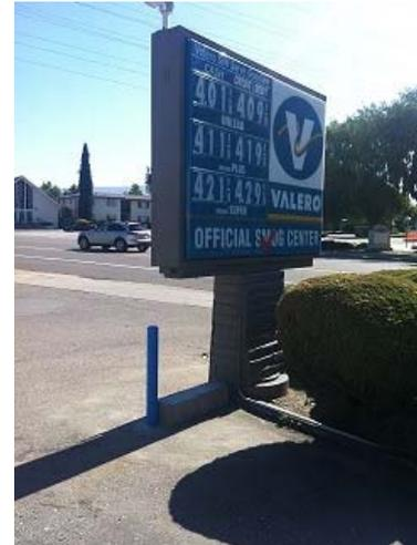
Oops... the building department missed this one. This before and after view shows an encroachment hazard along a path of travel with bottom edge of sign 40 inches above pavement. The sign was not lowered to less than 27 inches above pavement to comply with 2013 CBC Section 11B-307.2, instead a bollard was installed at the end of the sign and 8 inch height grouted masonry curb was installed below the sign to create detection for an individual using a cane.
