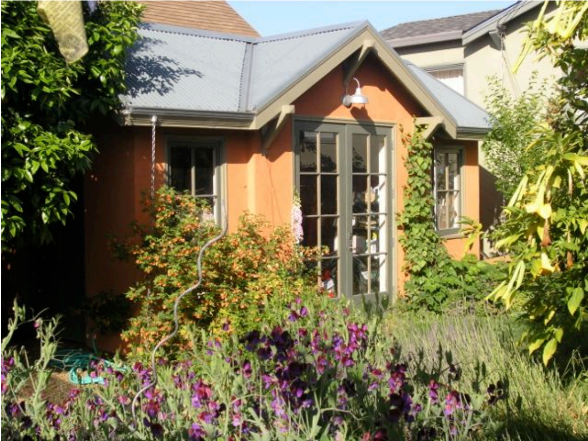
Figure 1-8. A detached workspace, James Avenue Live-Work Compound, Oakland, 2001. Thomas Dolan Architecture & Jennifer Cooper Designer.
