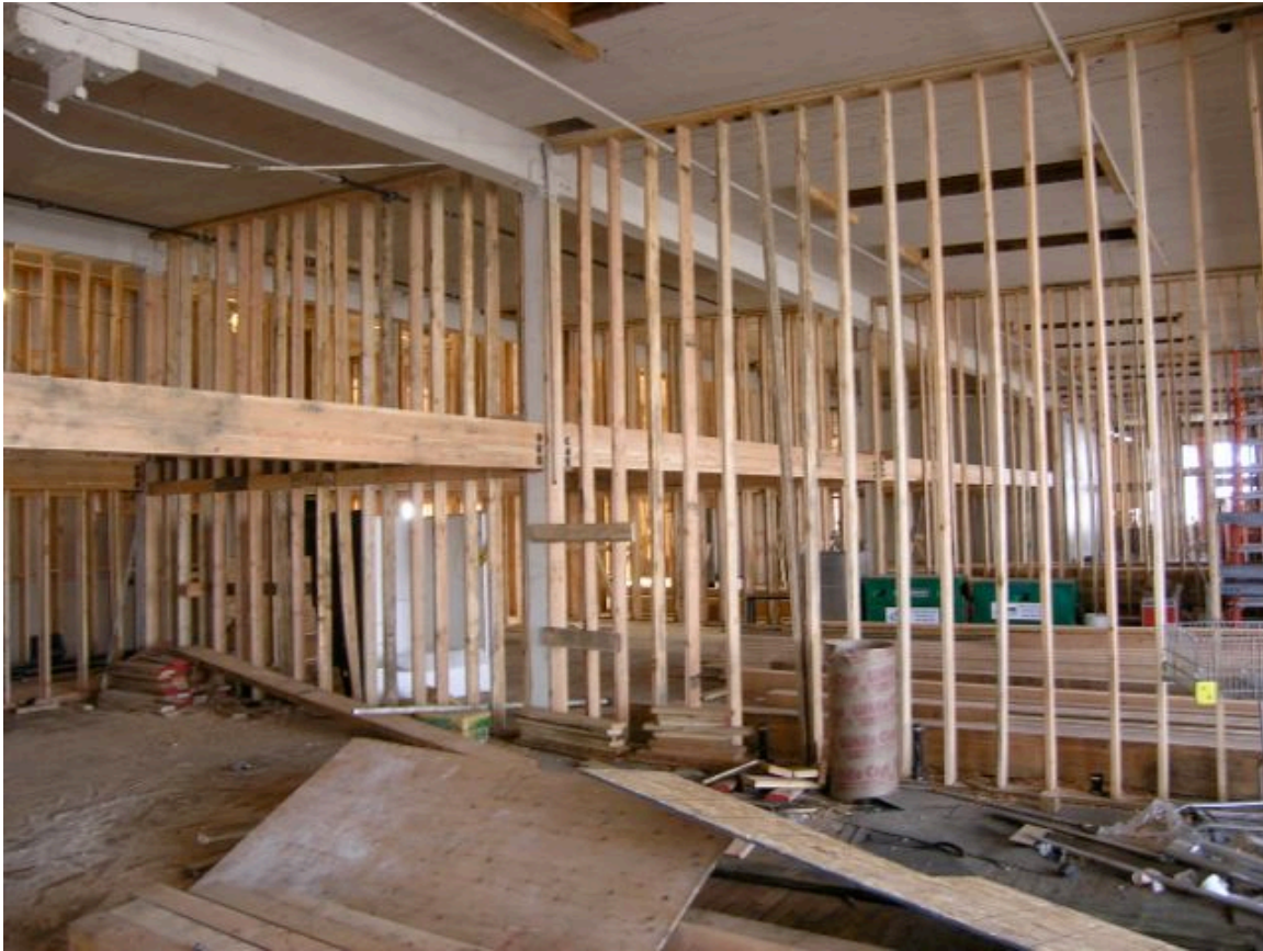
Figure 1-2 A large live-work renovation under construction. California Cotton Mills Studios, Oakland, 2006. Thomas Dolan Architecture.
